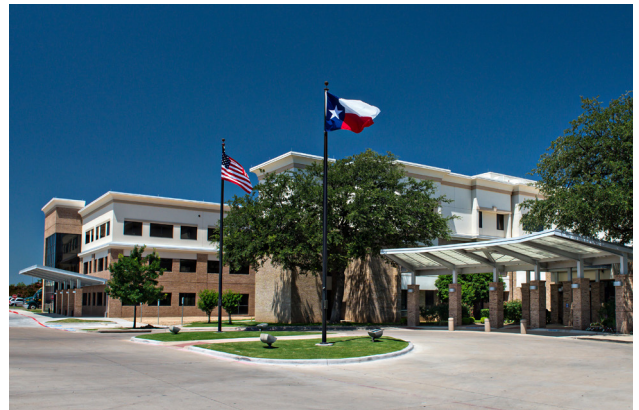
Lake Granbury Medical Center, Granbury, TX
